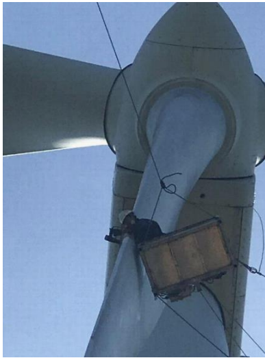
Figure 5. Wind Turbine Blade Human Inspection Method
